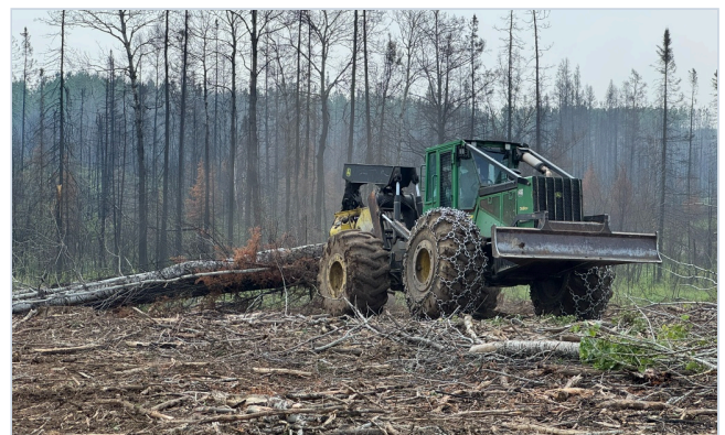
FIRE RECOVERY: Heavy equipment clearing timber and brush on a burn site following the Brimson Complex wildfires.
